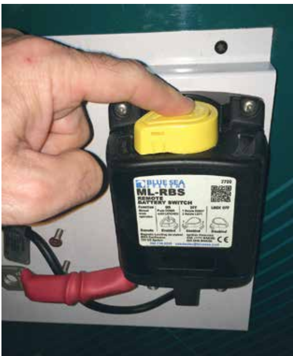
Main Battery Relay & Active Cell Balancer.
