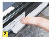
Apply foam tape all the way around the mainframe flange. Top corner of the window is a suitable starting point. Take particular care around the 2 radius corner. Cut off tape end at the starting point to form a continuous seal. Join foam tape, cleanly, as above. Apply bead of silicone to foam tape.
