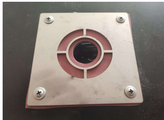
View of exhaust floor plate from below
