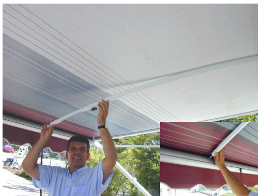
Extend out front telescopic section and fit spigot tip into hole in roller tube.
