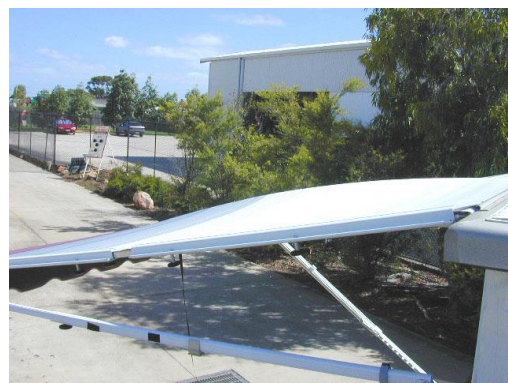
Shows Curved Roof Rafter in position.
