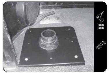
Using the Male to Male Coupler (Item 5), screw it into the tank. Place the Filler Cap (Item 2) onto the Male to Male Coupler and fully tighten. Make sure all componets are centerlized.
